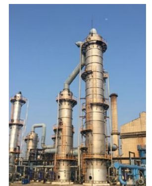
Facility that uses CO 2 capture technologies supplied by Carbon Clean Ltd.
