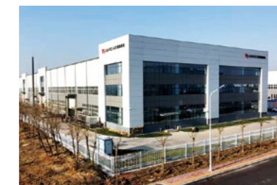
Marubeni Nisshin Feed Technology (Tianjin) Co., Ltd.
