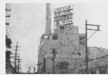
Manila Electric Company's generator No. 1 (Philippines)
