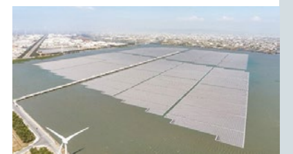
Floating solar power generation plant in Changhua, Taiwan
