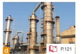
Image d: Facility that uses CO 2 capture technologies supplied by Carbon Clean Ltd. P.121
