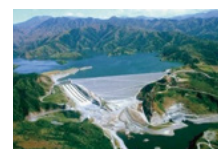
San Roque Hydroelectric Power Generation Project (Philippines)
