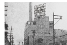
Manila Electric Company's generator No. 1 (Philippines)
