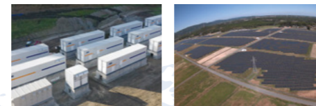
Energy Storage Systems Batteries
