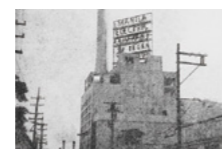
Manila Electric Company's generator No. 1 (Philippines)
