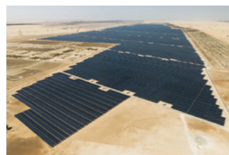
Sweihan Photovoltaic Independent Power Project
