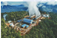
Rantau Dedap Geothermal IPP Project (Indonesia)
