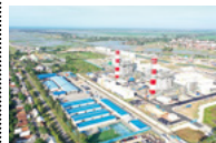
Jawa-1 Gas-to-Power Project Gas-fired power plant and floating storage and regasification unit (FSRU) (Indonesia)
