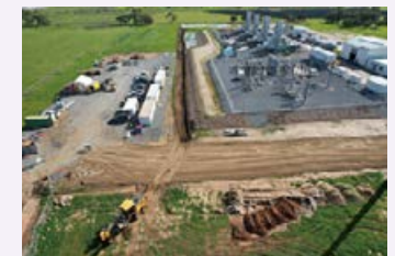
Demonstration facility under construction
