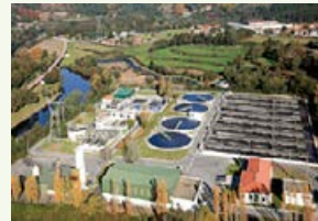
Water and wastewater services
