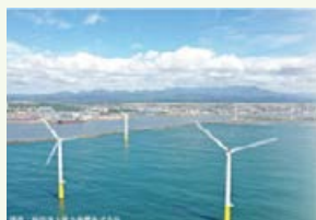
Offshore wind farm project at Akita Port and Noshiro Port (photo courtesy of Akita Offshore Wind Corporation)
