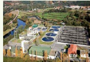
Water and wastewater services
