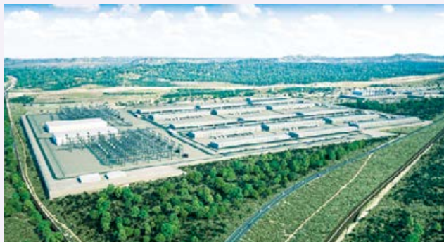
Image of hydrogen production site
