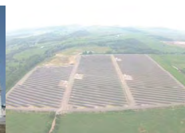
Tomakomai Yufutsu Mega-solar (Hokkaido)
