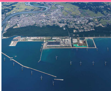
Offshore wind farm at Noshiro Port in Akita Prefecture (artist's impression courtesy of Akita Offshore Wind Corporation)
